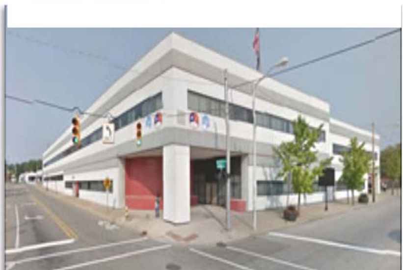
GCCARD ADMINISTRATION BUILDING
